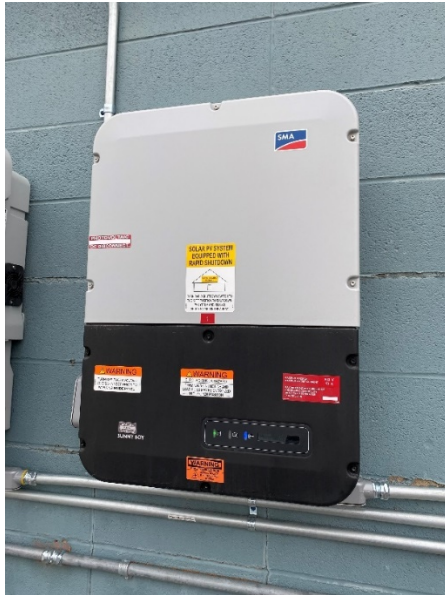
Figure 3: Example Picture: Inverter Installation on a Wall (Source: Luecken, 2023)
